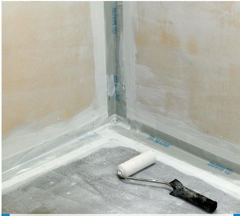
4. Apply a Mapegum WPS
