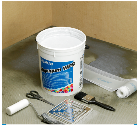
2. Prepare the tape for joints
