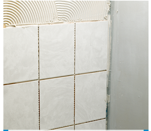
5. Apply grout and sealant
